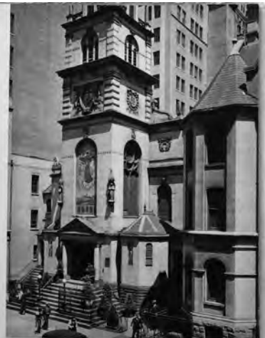
St. Francis of Assisi, on 17th Street between 6th Avenue and 7th Avenue. A small garden in the rear of the church is mentioned in the text.
